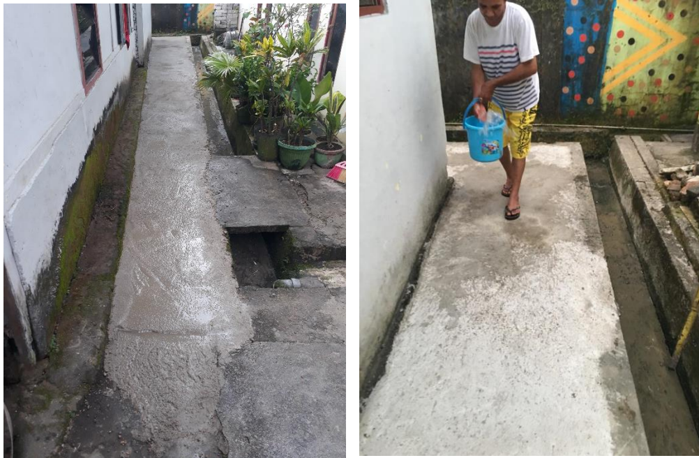
Gambar 3. Proses Perawatan/curing Beton Pasca Pekerjaan
